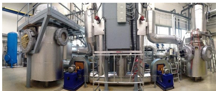
LOCA (Loss-of-coolant accident) device
