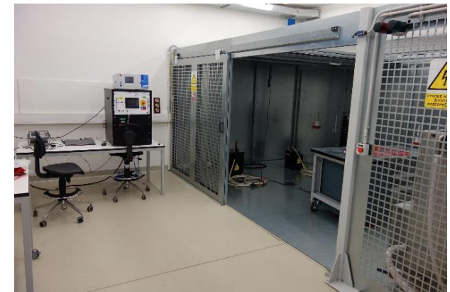
High voltage laboratory
